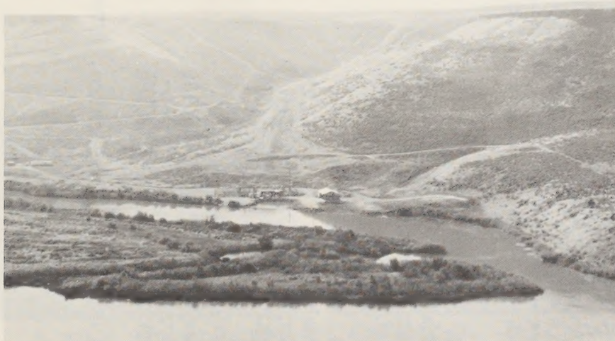
FIGURE 1-5. Aerial panorama of pump station located on a side channel of the Snake River. A buried penstock ascends the hill behind the station to deliver irrigation water to the bench high above the river.
